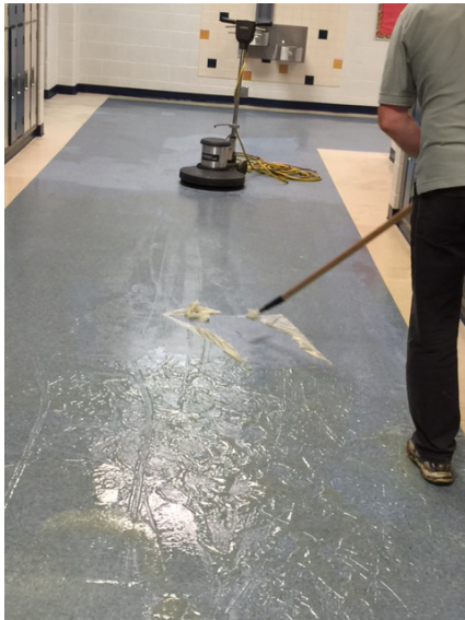
Shred being tested on a school hallway. The sales consultant lifts dozens of layers with a floor scraper thanks to the new gel product.
